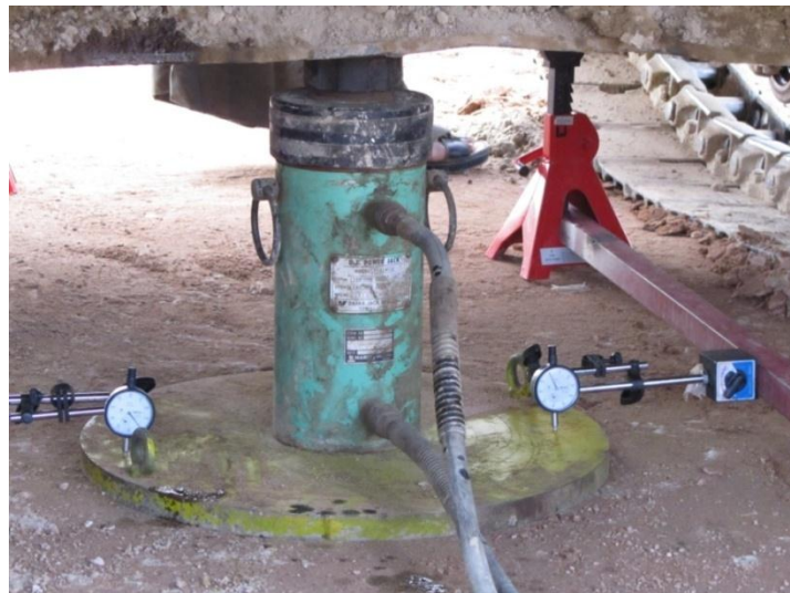
Plate (1): Plate Bearing Test for Location of Point (1)
