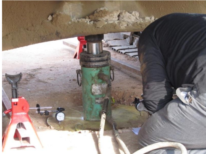
Plate (2): Plate Bearing Test for Location of Point (2)
