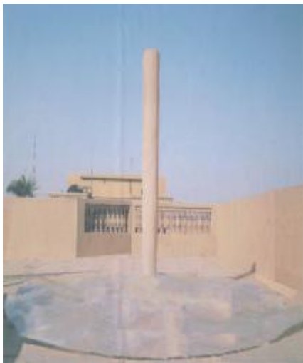
Figure (3) Photo for the solar chimney prototype
