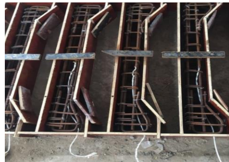
c- Installing thermocouples to the steel bar
