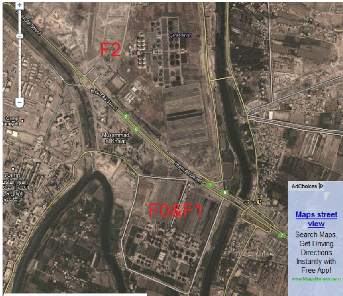
Fig(1) Al-Rustamiya wastewater treatment plant.
