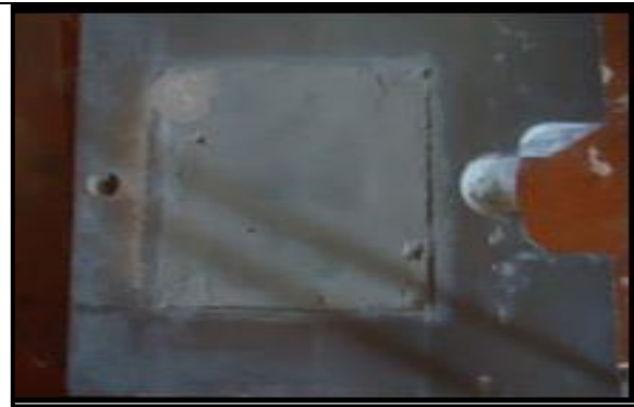
Figure 3. Concrete Interface surface
