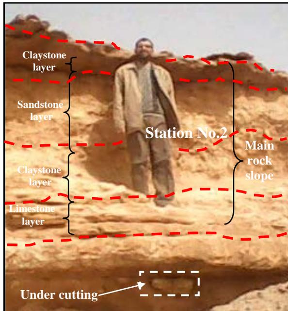
Plate 2: The slope of station No.2. Front view showing rock fall, photo direction SE
