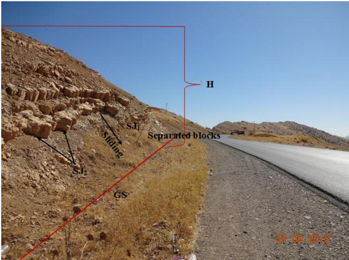
**Figure 4-** Side view of the slope in station No.2 in Kalkasmag-Koysinjaq road shows height of slope SJ1, SJ2, bedding plane, and separated blocks.
