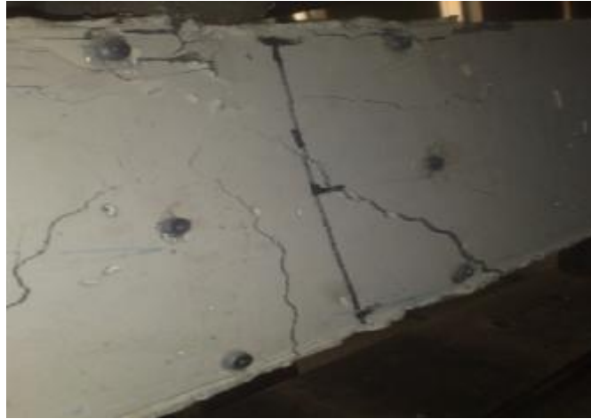
Figure (5) Flexural failure.
