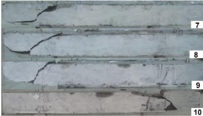
Figure (2), Crack pattern of reinforced concrete beams
