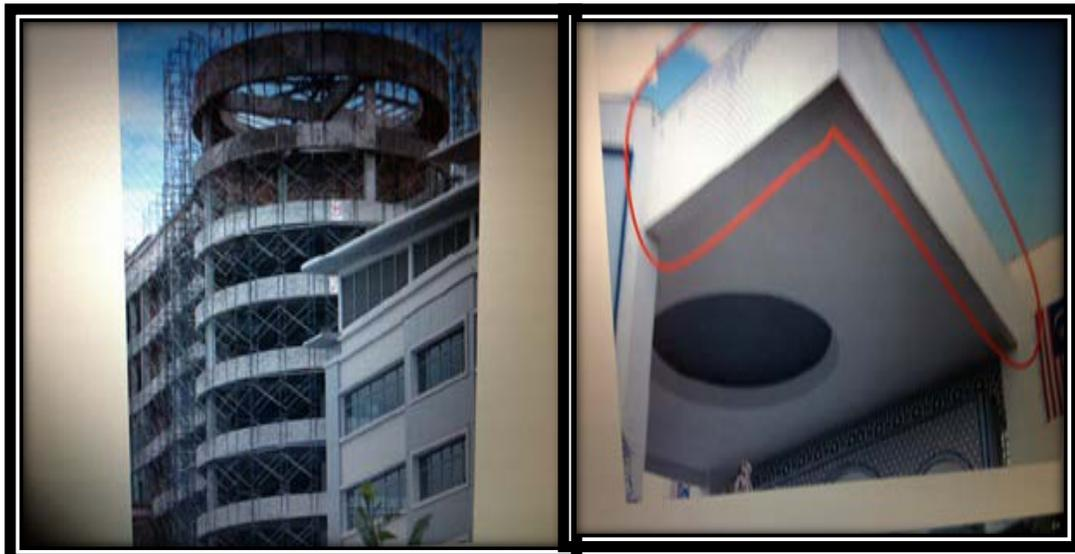
**Fig. (2): Reinforced Concrete Members Subjected to Torsion.**<sup>[3]</sup>
